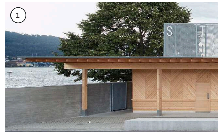
Timber frame external with butterfly roof
