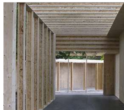
ST1.1/3: Efficient low carbon off site timber frame superstructure
